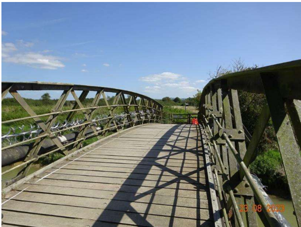
Figure 22: View looking east shows footway surfacing.
