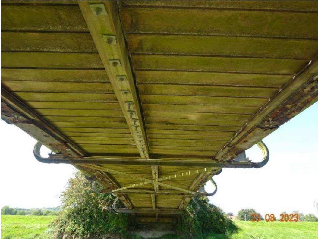
Figure 13: Timber deck elements, following 2013 refurbishment.
