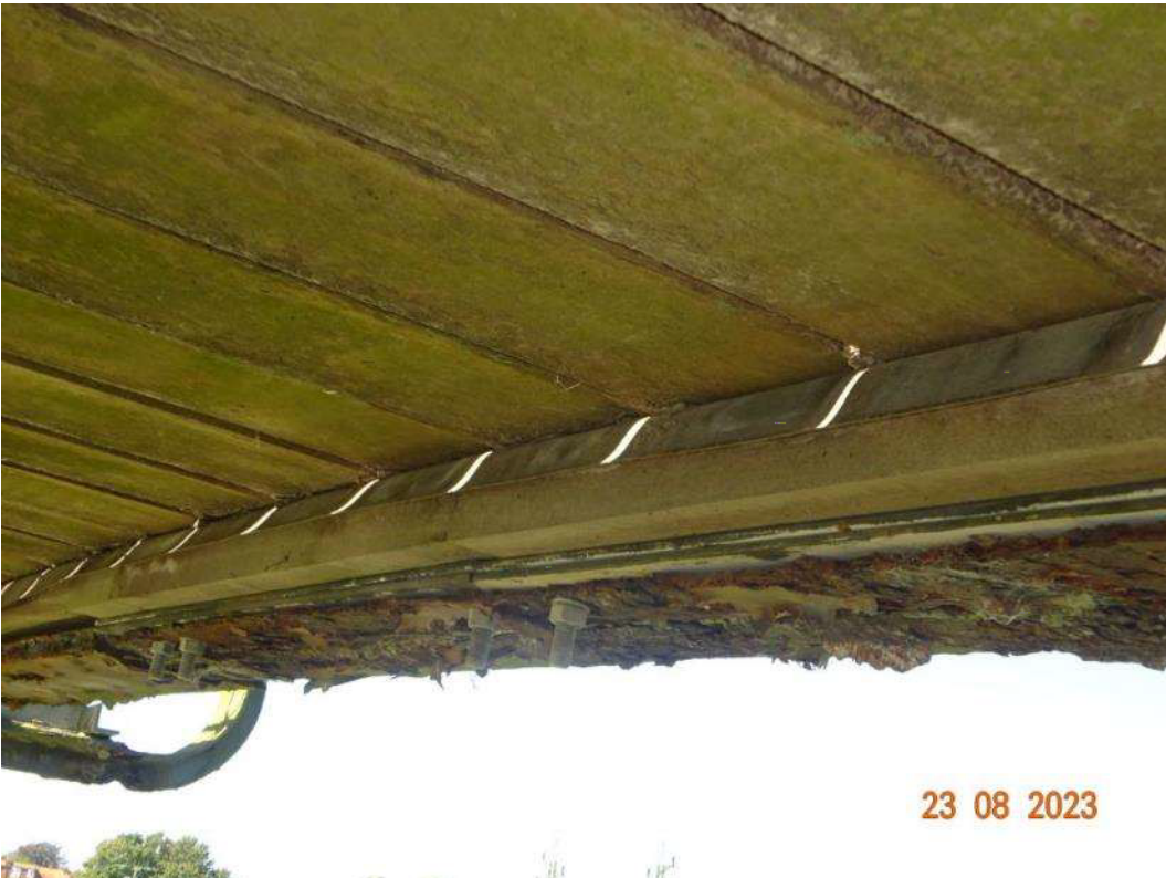
Figure 14: View of timber deck configuration with bottom chord.
