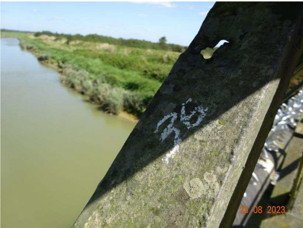
Figure 10: Historic perforations within diagonal bracing (north)
